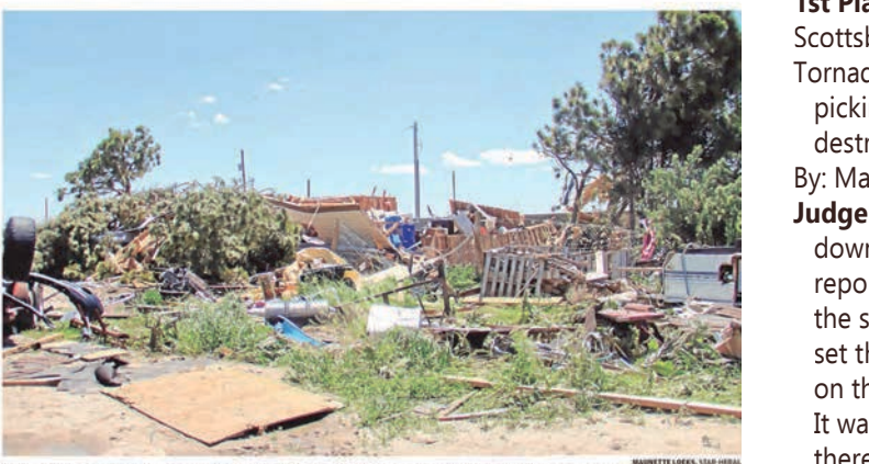
What remains of the Wilson family's home and garage can be seen on Saturday, June 24. Their home along Highway 26 east of Scottsbluff was destroyed by a tornado that tore through the area on Friday, June 24. Photo by Nathan Arneal.
